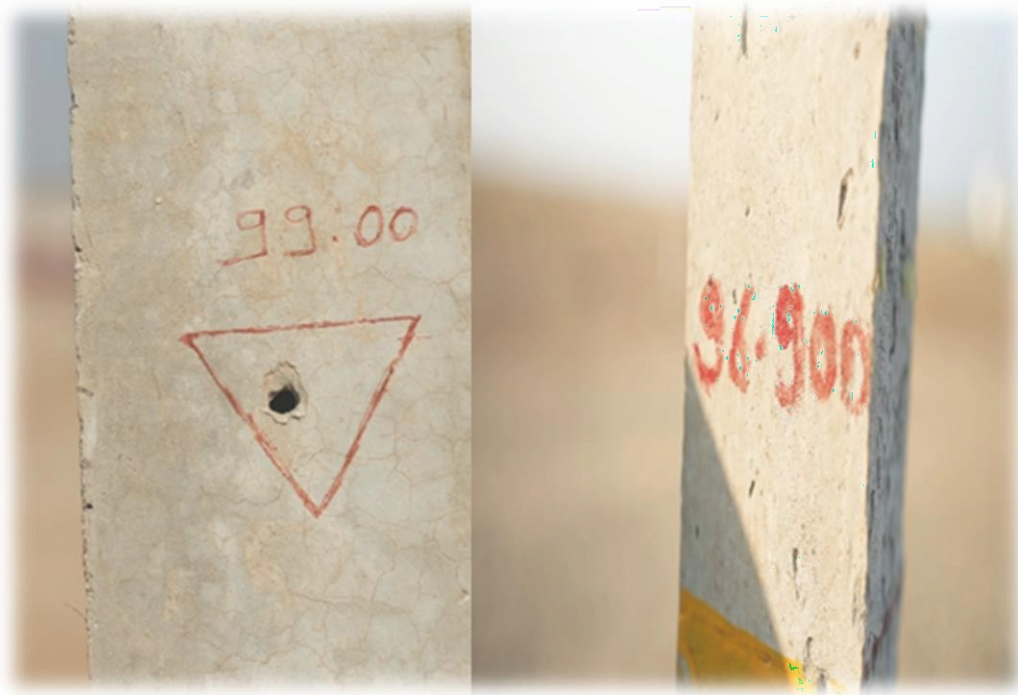
Photo of actual elevation measurements Plinth level 1 – 99.00 Plinth level 2 – 96.90 Elevation Difference- 2.1m
